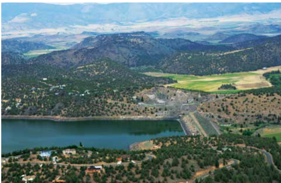
Water captured from the Shasta river is stored in Dwinnell Dam. The Shasta River once provided much of the cold water coho salmon need, but in 2009, only 9 coho made it back. Water captured from the Shasta River is stored in Dwinnell dam, pictured here.
