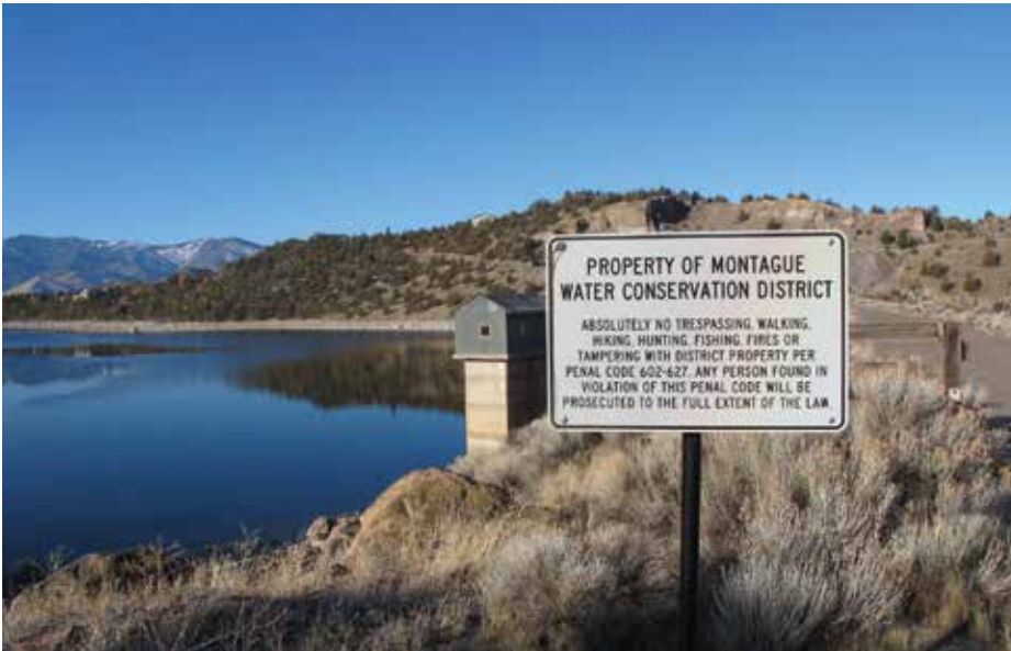
Close up view of Dwinnell dam on the Shasta river. For the first time, the Montague Water District will be required to release water for fish populations.
