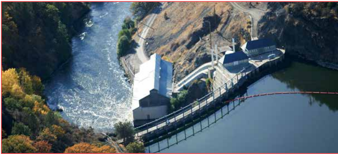
Blocking fish for nearly a century, PacifiCorp's Copco 1 Dam is so antiquated it would be cheaper to remove than to update. Photo by KRK/Northern California Aerial Photography.
