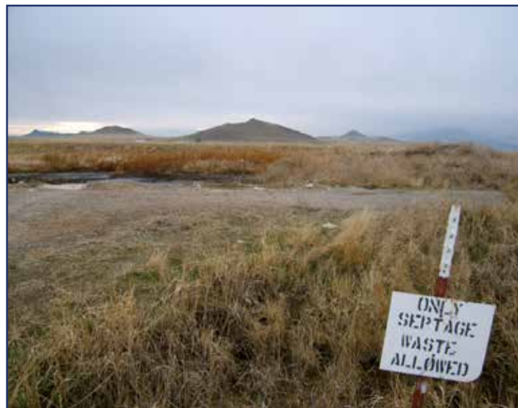
Siskiyou County received a warning this winter from the California Water Board regarding this unlined - and unregulated - pit for the storage of raw sewage.
