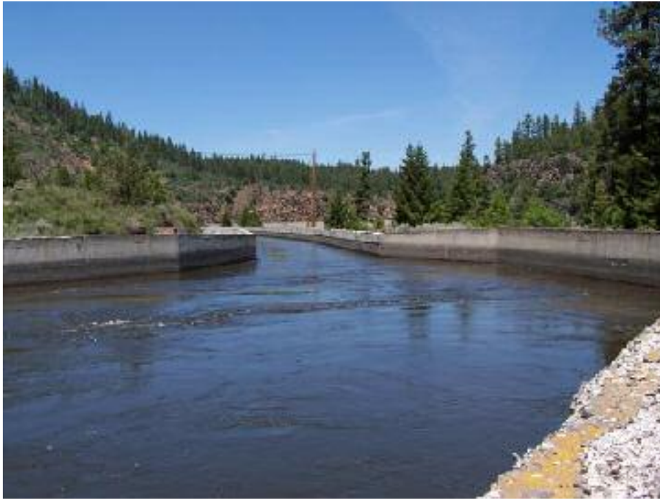
Figure 4. The canal that carries water from J.C. Boyle to the powerhouse. Photo by Katherine Pedery ( http://www.pelicannetwork.net/salmon.boyle.htm ).
